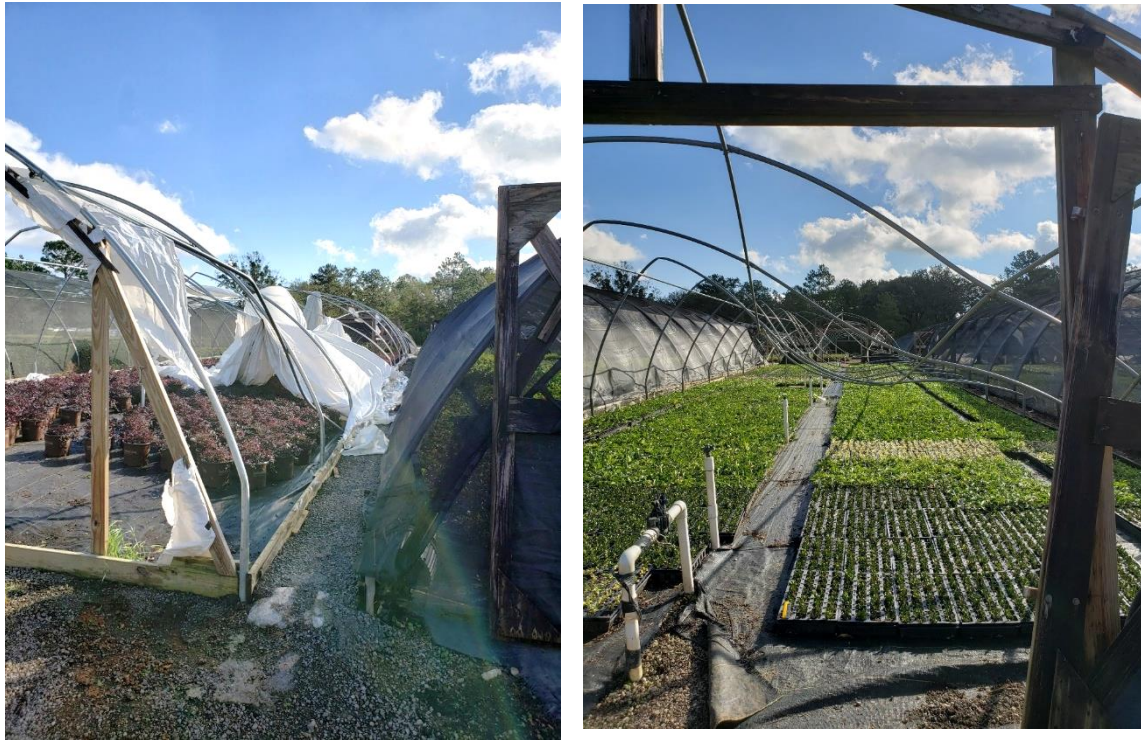
Figure 8. On 24 October 2020, Hurricane Zeta destroyed eight Quonset houses.
