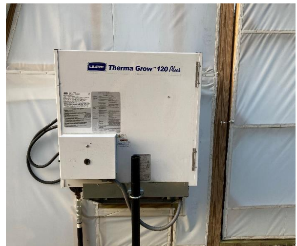
Figure 22. (left) Covering greenhouses with 50% opacity plastic for winter protection, and (right) outdoor mounted, direct fire, forced air heat for high efficiency heating.
