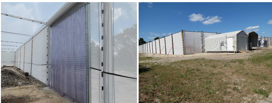
Figure 3. (right) Citrus under protective screen (CUPS). (left) Steel roll-up door with a second plastic strip door, and (right) citrus can be grown under protective screen structures for fresh-fruit production in order to exclude the Asian citrus psyllid (ACP, Diaphorina citri ) vector of huanglongbing (HLB), or citrus greening disease, and thereby produce disease-free healthy fruit. While CUPS may be economically feasible for some fresh-market citrus crops, over 90% of Florida citrus is for juice production, so a CUPS system is not economically sustainable. https://edis.ifas.ufl.edu/publication/HS1304 Credit: Arnold W. Schumann, UF/IFAS.
