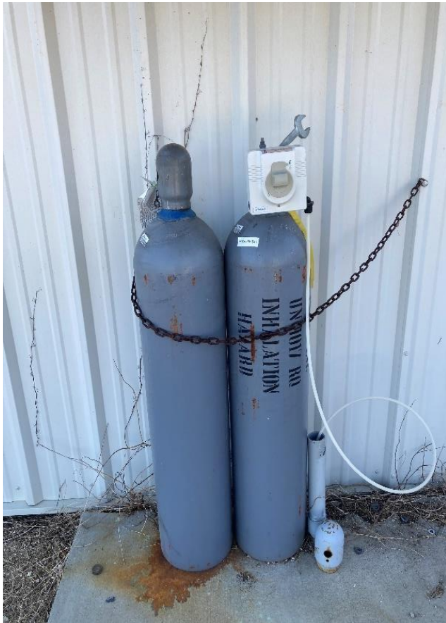
Figure 17. (top left) Interior view of pump house, (top right) a Yardney sand filtration system with automatic backflush, (bottom left) chlorine gas cylinders with a regulator, and (bottom right) a Wallace and Tiernan ® S10k gas feed chlorine metering system.
