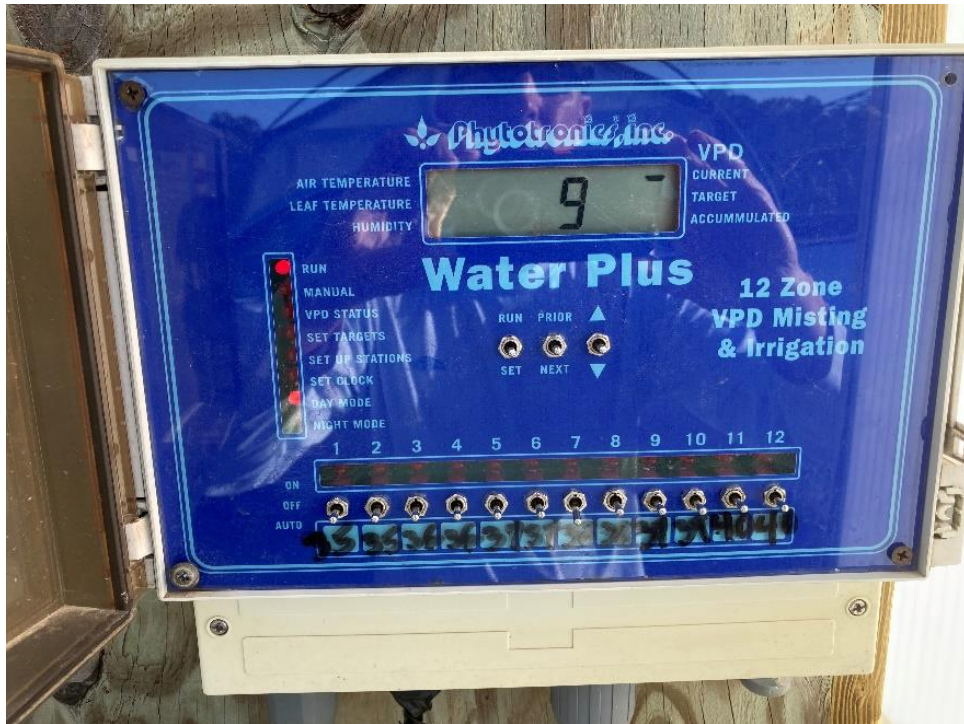
Figure 14. Phytotronics 12-zone vapor pressure deficit (VPD) controller.
