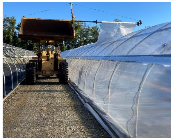
Figure 12. (left) A 9x44 m (30x145 ft) greenhouse covered with 50% shade cloth and 2 m (6-ft) plastic side curtains. (right) Applying a double layer of clear plastic to greenhouse using boom attachment.
