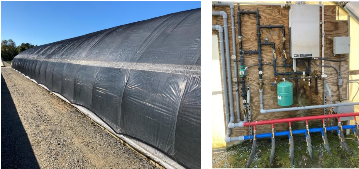
Figure 13. (left) Greenhouses converted for cool season propagation, and (right) wall mounted propane fired hot water heating system.
