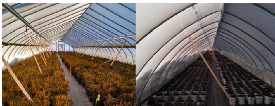
Figure 3. Placement of supports to prevent snow load damage.
